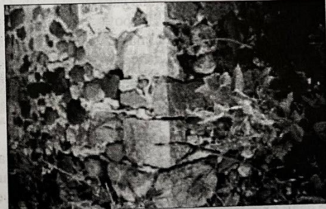
Square stone silo, Waukesha County.
